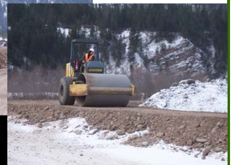
Compacting the berm
