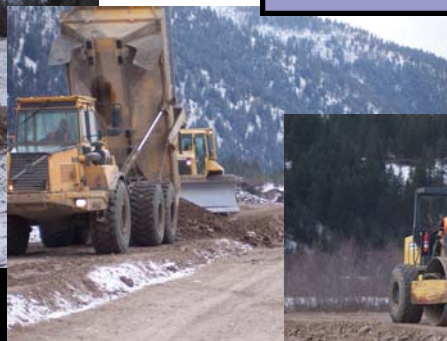
Placing berm material in 12" layers
