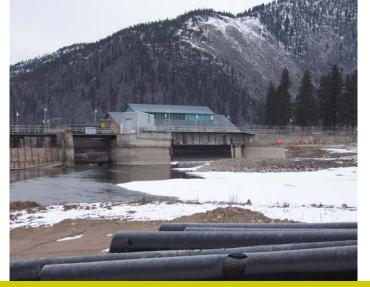
The Milltown Dam - looking downstream (west) from on top of the new Clark Fork River flood berm. In the foreground are rolls of the black geo-tech fabric used in berm construction.
