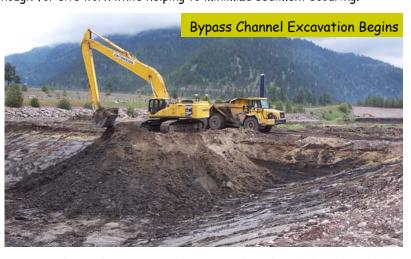
averaging 4,000 cubic yards per day. To control erosion, the sides of the channel will be lined with "reno mattresses" (wire bound rocks in the shape of a mattress). The bottom of the channel will be rough enough to provide the "loafing" areas necessary for fish passage. The bypass channel is a critical element in minimizing downstream impacts of the project on fish and other aquatic life, as well as on downstream users.
