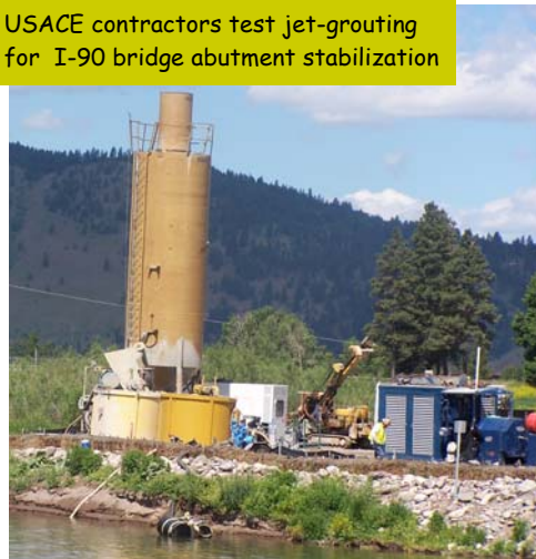
USACE contractors drill holes for I-90 bridge stabilization
