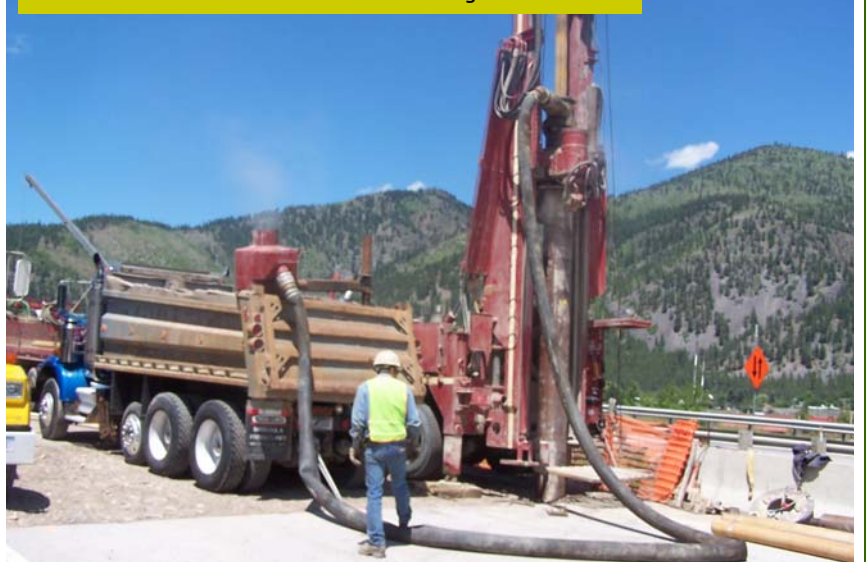
USACE contractors drill holes for I-90 bridge stabilization
