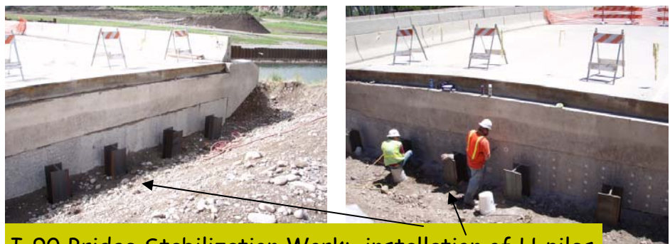
I-90 Bridge Stabilization Work: installation of H-piles
