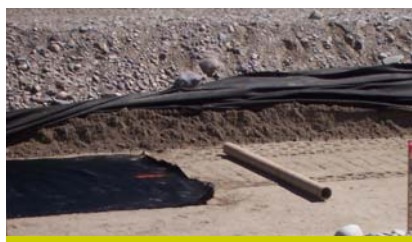
Rail spur base covered with geo-fabric
