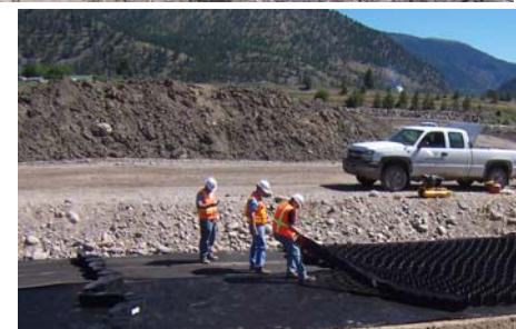
Rail spur base covered with geo-fabric
