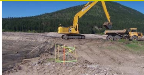
Clark Fork River Bypass Channel excavation— east end
