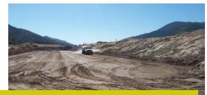
Bypass Channel - as seen from the bottom of the new channel; water truck actively controlling dust on-site
