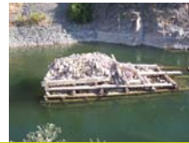
Timber cribs being removed from BFR
