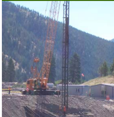
Installation of the rail bridge over the Bypass Channel
