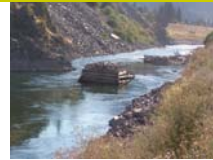
Timber cribs being removed from BFR
