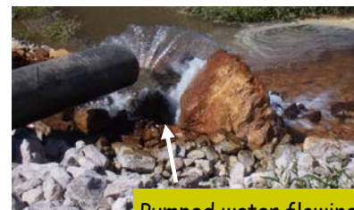
Pumped water flowing into Sedimentation Pond. Note iron-stained rocks.
