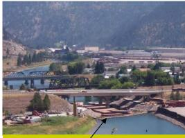
Red "flexifloats" (barges) are placed in the Blackfoot River by USACE's contractor in preparation for stabilization work on the I-90 Bridge Center Piers.
