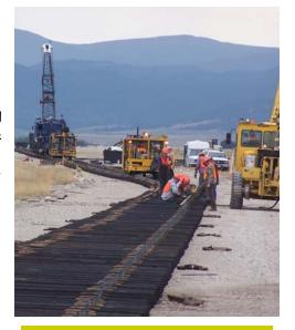
Montana Rail Link workers installing track to the BP/ARCO repository at the Anaconda Smelter Superfund Site.
