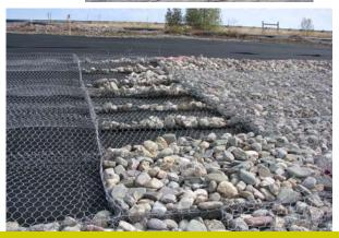
Wire cages filled with rock to form base of the reno mattress; a wire cover is then added to complete the mattress and line the Clark Fork River bypass channel.
