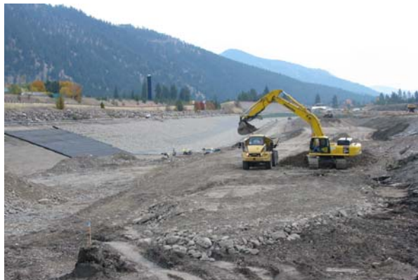
Workers continue to build the Bypass Channel Berm. When the bypass channel is complete, the Clark Fork River will be re-routed through this clean channel, effectively isolating the contaminated sediments from the active river. The channel can withstand a 100-year flood.
