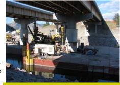
Drilling shafts under the I-90 bridges on the Blackfoot River to ensure bridge stability after the Milltown Dam is removed.
