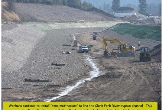
Vorkers continue to install "reno mattresses" to line the Clark Fork River bypass channel. This week, workers began installing the liner on the bottom of the bypass channel.
