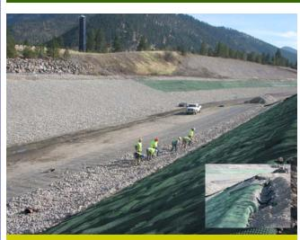
The Clark Fork River bypass channel — 4,000 feet long and built to withstand a 100-year flood event — is nearing completion. Workers are seen lining base and south side of channel. *Insert:* Anchoring the Turf Reinforcing Mat into the berm.
