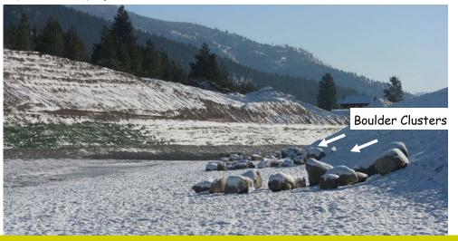
View from the bottom of the bypass channel, looking upstream (to the east). The bypass channel is 4100 feet long and 100 feet wide at the base. Boulder clusters will aid in fish passage. It will be completed in January 2008.
