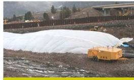
"Tent dryer" used to warm up soil to allow construction of the berm on the south side of the bypass channel.
