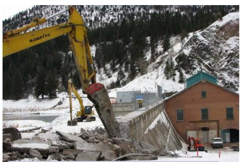
Removal begins of the right (north) abutment wall of the Milltown Dam Structure, 1/15/08.
