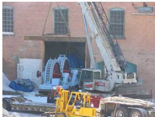
Preparing to load generators, 1/23/08
