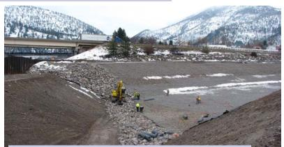
2/12/08, Tying bypass channel liner into the grade control structure at the bypass channel outlet. In a few weeks, the Clark Fork River will be diverted into this channel, isolating the river from the contaminated sediments.
