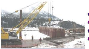
Removing barges from the Blackfoot River, 2/12/08. The 90 barges created a work platform during I-90 bridge mitigation.
