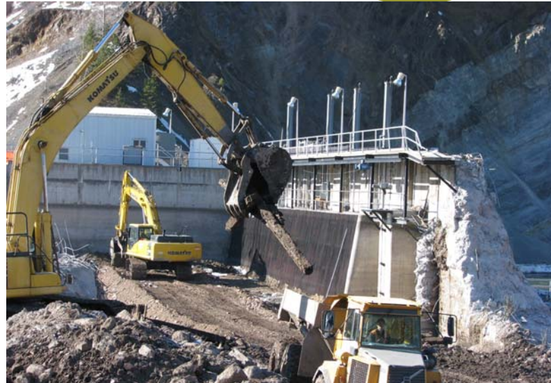
Forebay wall is removed; timbers are recovered from original timber-crib dam, 2/19/08
