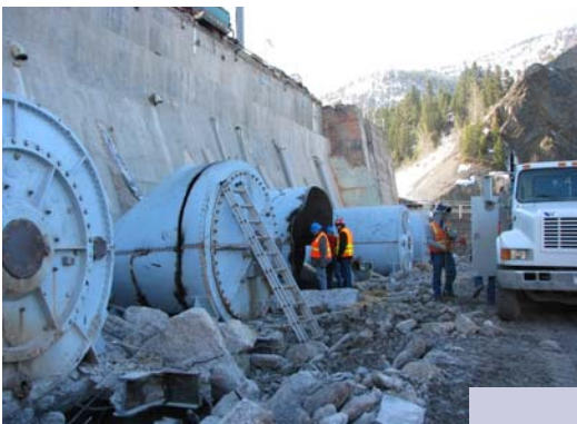
Penstock removal at the Powerhouse, 2/19/08
