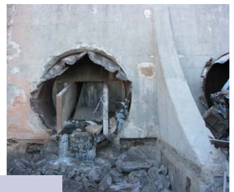
Penstock removal at the Powerhouse, 2/19/08
