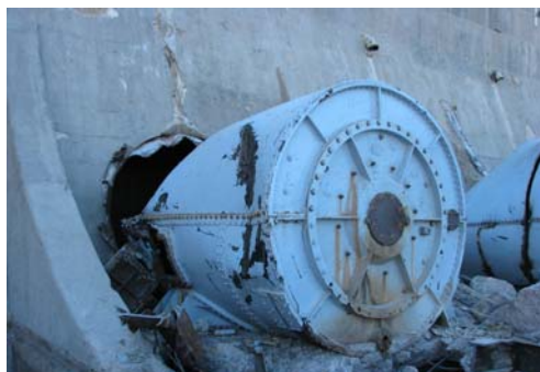
Penstock removal at the Powerhouse, 2/19/08
