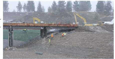
Looking downstream from the Bypass Channel Inlet: Lining the Clark Fork River bypass channel. The bypass channel should be complete by the end of next week.
