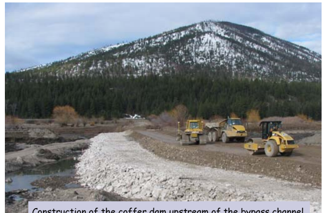
Construction of the coffer dam upstream of the bypass channel.
