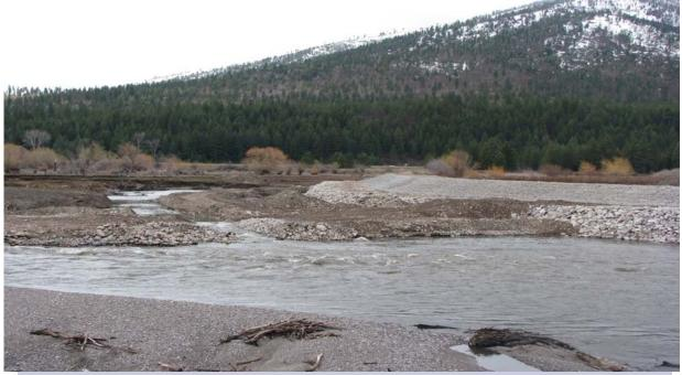
Shown on center Right is the finished upstream dike blocking of the CFR at head end of bypass channel. Deer Creek is entering bypass channel at center left.
