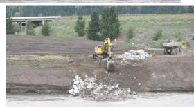
5/21/08: Building the "Flow deflector" to keep clean soils from eroding from north side of the Clark Fork River above the Dam.
