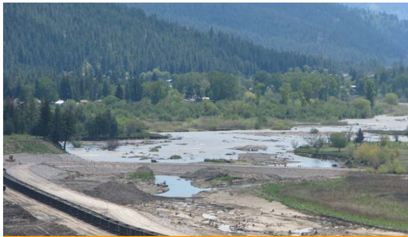
Upstream of the cleanup area the Clark Fork River is changing as stream material is eroded and re-deposited. The former river channel is drying up behind the diversion dike.
