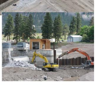
**Continue excavating sediments and loading 45 rail cars each day**. To date, **955,076 tons** (830,500 cubic yards) of sediment have been hauled to the Anaconda Smelter Superfund Site for use in site reclamation.
