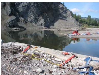
Pool below Dam spillway, 9/2.
