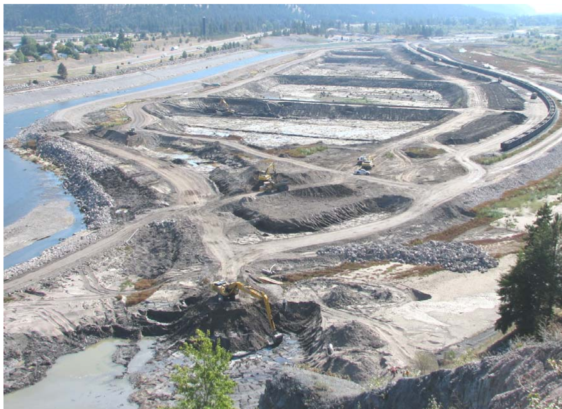
View of the Milltown Project area showing bypass channel, cells of excavated sediment, and the rail cars being loaded for transport. All photos by Keith Large, DEQ, 9/16/08.
