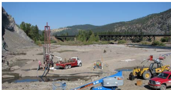
The photo above shows sediment dewatering continuing downstream of the former dam spillway.
