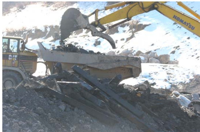
Removing the final remnants of the Milltown Dam spillway,
