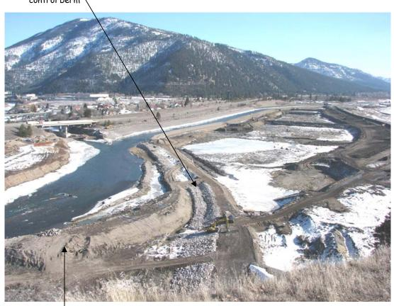
Spillway coffer dam that will be breached in March 2009. At that point, the joint Clark Fork and Blackfoot River channel will flow along the base of the Milltown bluff (not visible from this view). Much of the material on the far side of the spillway area (including portions of the divider block) will be removed before high flow this spring. Photo taken 2/3/09.
