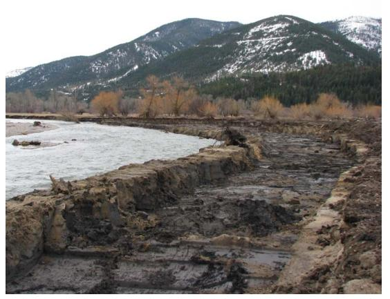
The photo above (3/3/09) shows the initial removal of contaminated sediments upstream of the remedial project area (Area 4) to prevent them from scouring during spring high flows. Preventative measures such as these reduce downstream river and fisheries impacts. If all goes as planned, up to 100,000 tons of material could be removed by April 2009.
