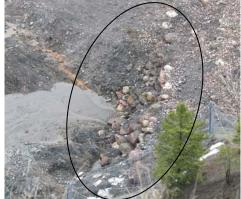
Grade control structure as seen from the bluff. When the de-watering pumps below the former spillway are turned off, this area will flood and the structure will no longer be visible. The "hole" is expected to fill in with cobbles and gravel during this spring's high flow.
