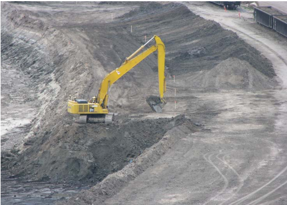
Excavating contaminated sediments from along the rail loading pad.
