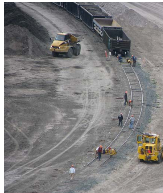
MRL beginning to pull the on-site rail line.
