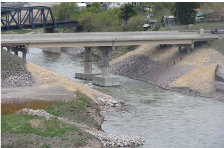
Newly seeded banks under the I-90 bridges.
