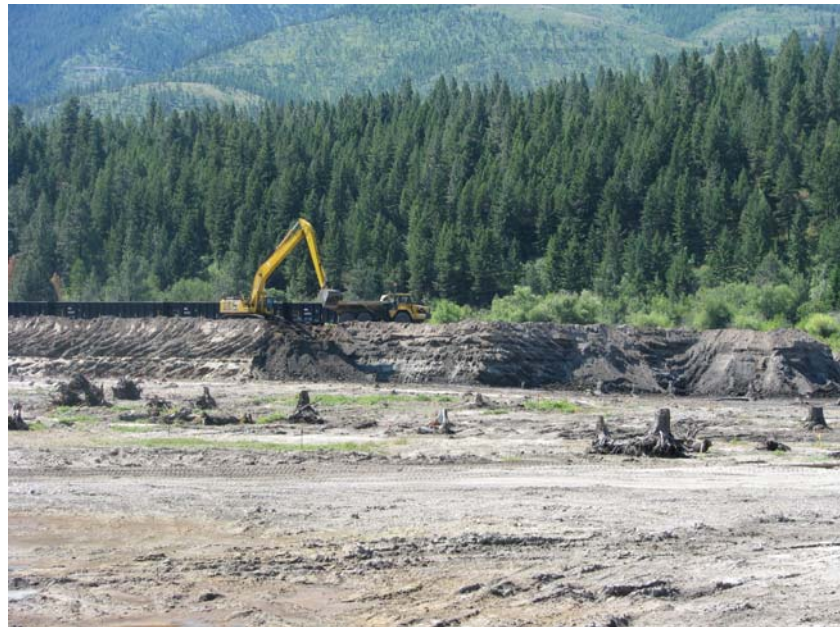
Excavating sediments from along the bed of the rail spur.
