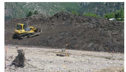
Stockpiling pre-dam native soils for later use in Site restoration.
