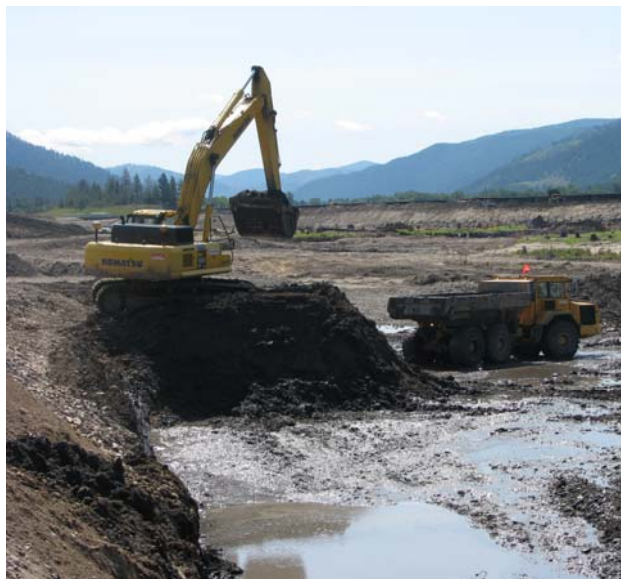
Removing Buried A-Horizon Soils from Area 2 – the location of the new Clark Fork River channel. These are pre-dam native top soils.
