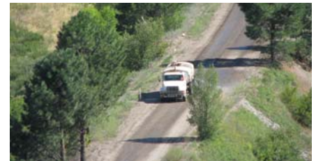
Water truck spraying haul roads to control dust on-site, 8/4/09.
