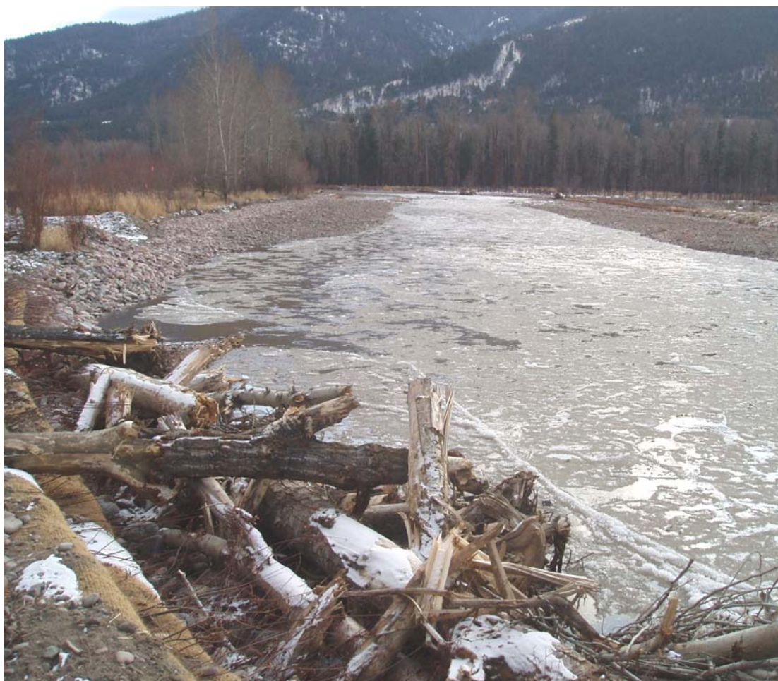
December 2009: Newly finished upstream channel of the Clark Fork River channel (Doug Martin photo).
