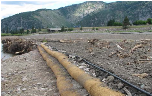
Photo at left shows the completed bank treatment along the new Clark Fork River channel — planted willows with irrigation.
