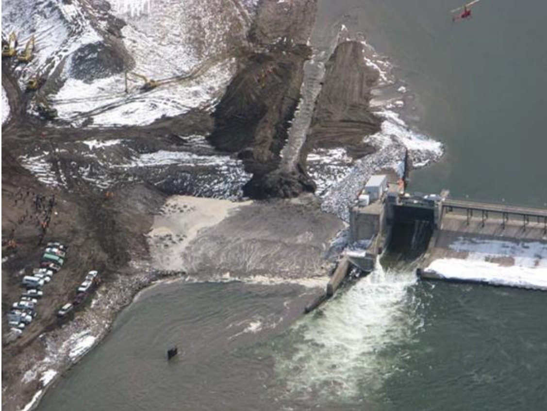
The photo above was taken by Judy and Gary Matson, West Riverside residents and members of the organization Friends of Two Rivers. It shows an aerial view looking upstream just after noon on the day of the dam breach, as water flowed into a narrow channel built to initiate the breach. Water flowed through the area previously occupied by the dam's brick powerhouse, adjacent to the dam's spillway.
