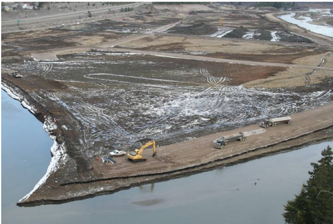
The photo above shows the reservoir sediments from the bluff above the dam on the south side of the river. Major construction activity at the site includes construction of flood control berms
