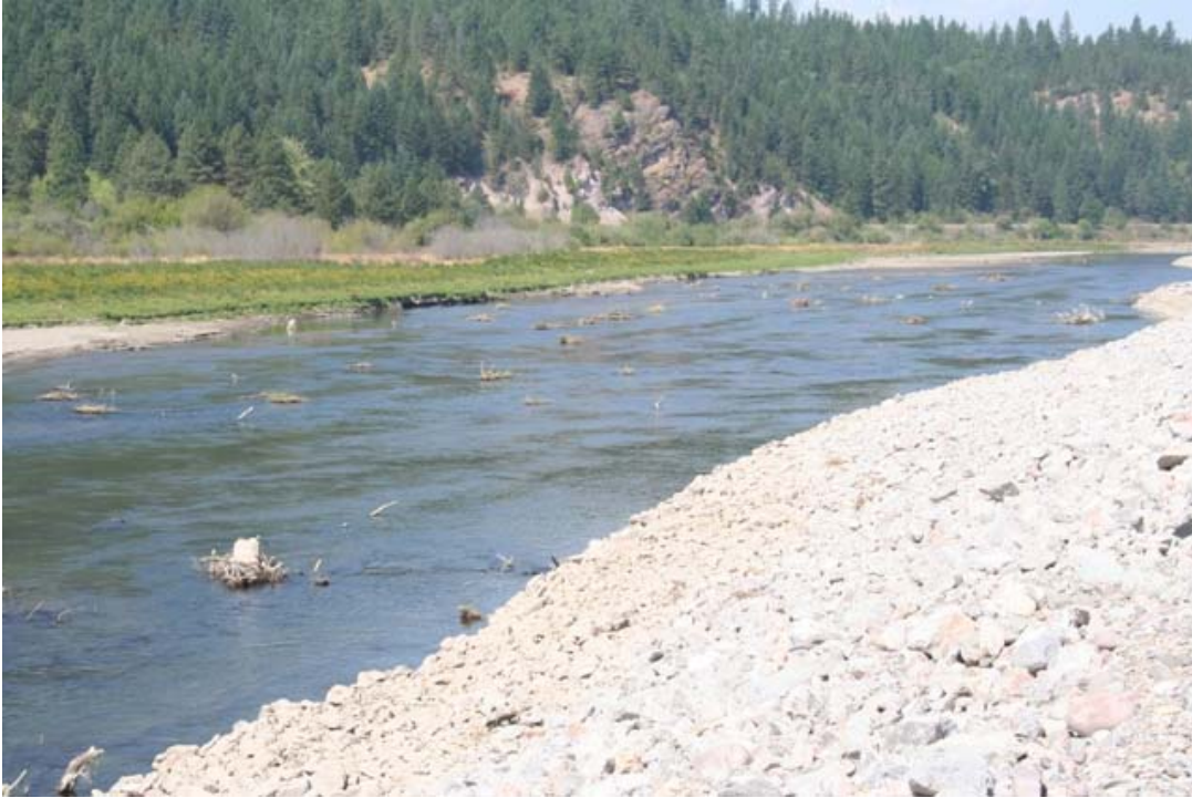
This photo shows another view of the stumps in the channel, taken from the flood berm in Envirocon's construction area.
