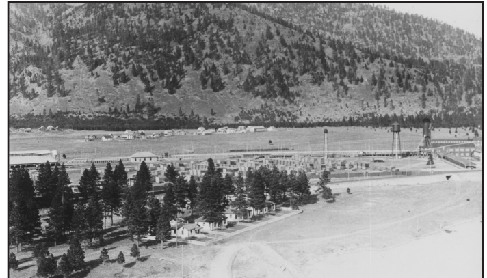
The settlement of West Riverside is shown in the background in this 1915 photo. Laborers who lived there owned their own property and homes. On the left are the houses of power plant employees. Also in the photo is the Western Lumber Company. Jack L. Demmons Photo Collection.
