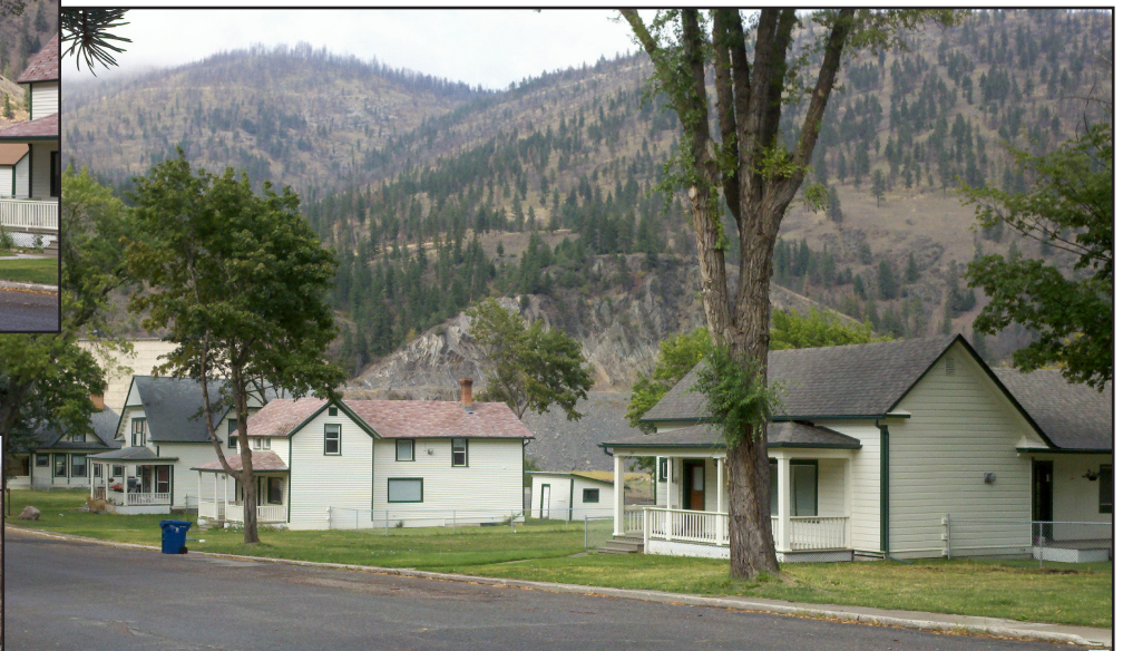
White House Lane, 2013. House 9 in foreground.
