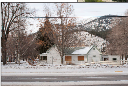
Mrs. Dix would be happy to see her house restored. House 9 in 2012 before restoration.
