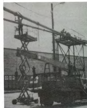
PNEUMATIC CONSTRUCTION, INC. Chip Pipe Installation and Repairs
