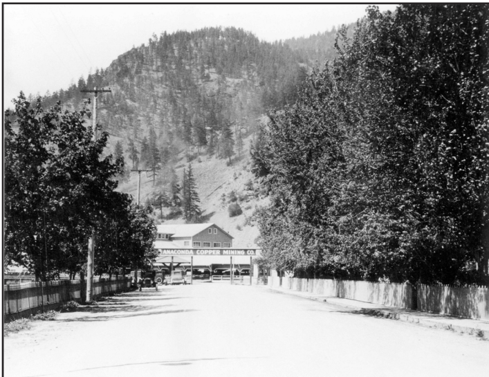
The original mill entrance
